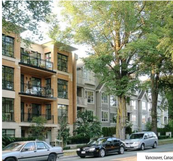
BOTTOM Modulated façade establishes vertical proportions that divide the mass of the building into bays; horizontal balconies that reduce the scale of the building's proportions create a well-articulated elevation Image Credit: Vassilena Sharlandjieva via www.ubyssey.ca
