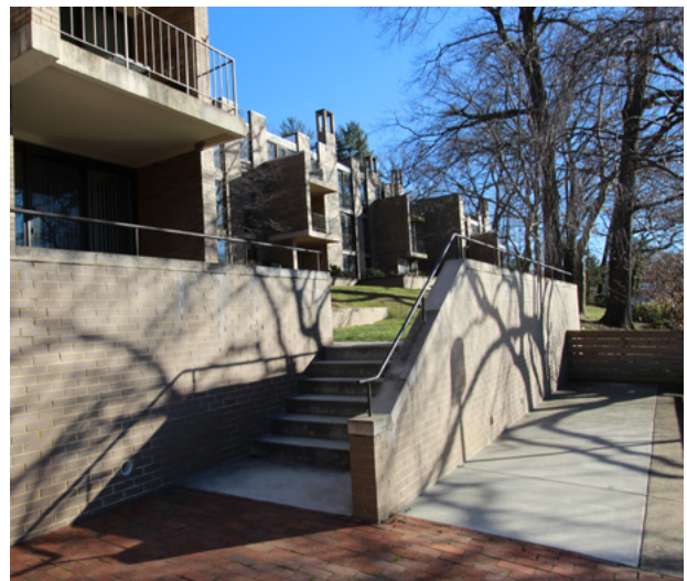
Exterior steps and retaining wall.
