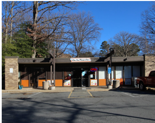
Former Garden Shop.
