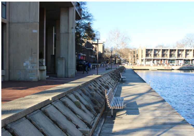
Wood benches and concrete walls.
