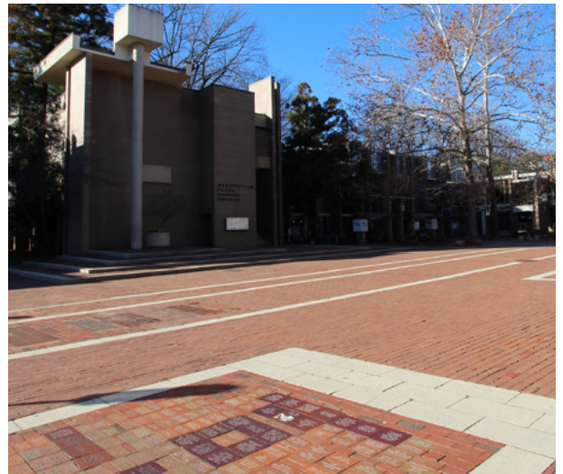
Red brick with concrete pavers.
