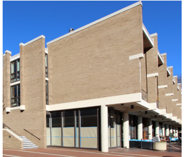
Brick cladding with concrete trim; overhanging upper story supported by cylindrical column.
