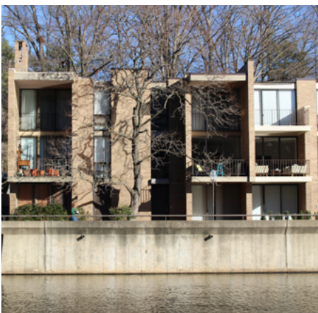
Concrete retaining wall along east edge of inlet.
