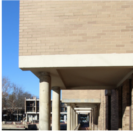
Buff brick with contrasting white concrete.
