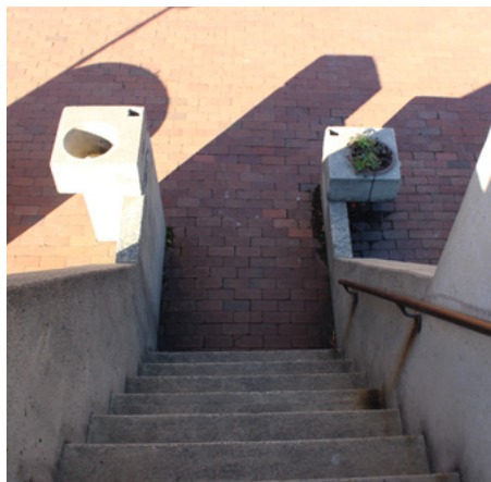
Concrete stair structure with integrated planters.
