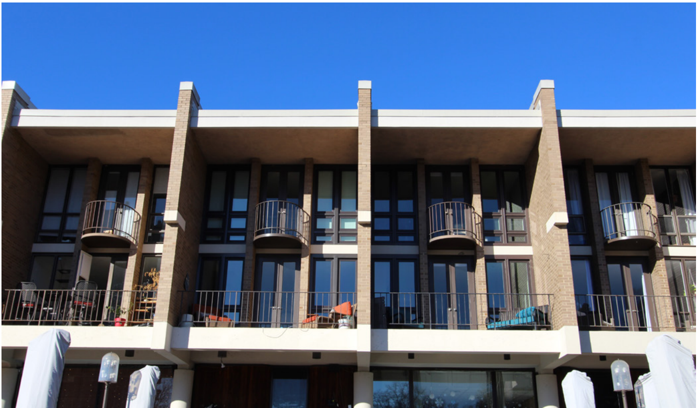
Detail of second- and third-story balconies overlooking Washington Plaza.
