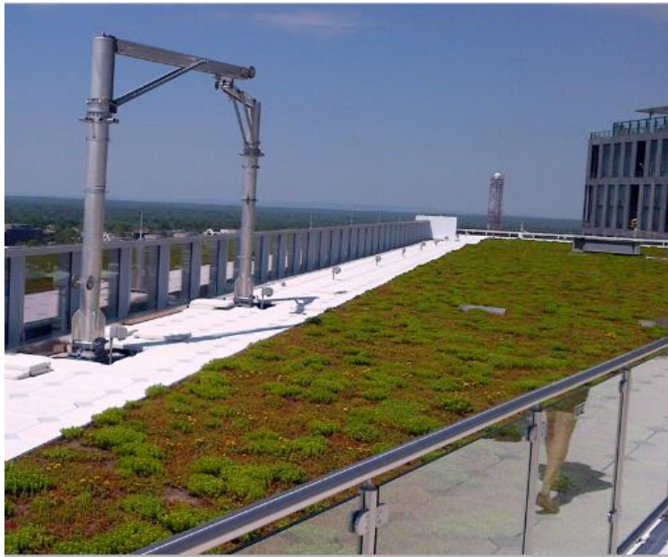
Extensive green roof at Tysons Corner Center
