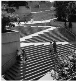
Figure 37- Integrated ramp and stair Source: https://st1le.files.wordpress.com/2012/04/webstramps.jpg
