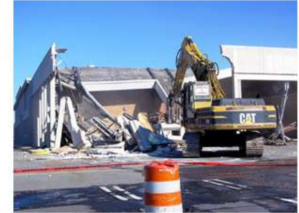
Demolition work in Summer, 2013
