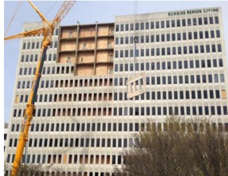
Removal of Precast Façade - 7900 Westpark Drive
