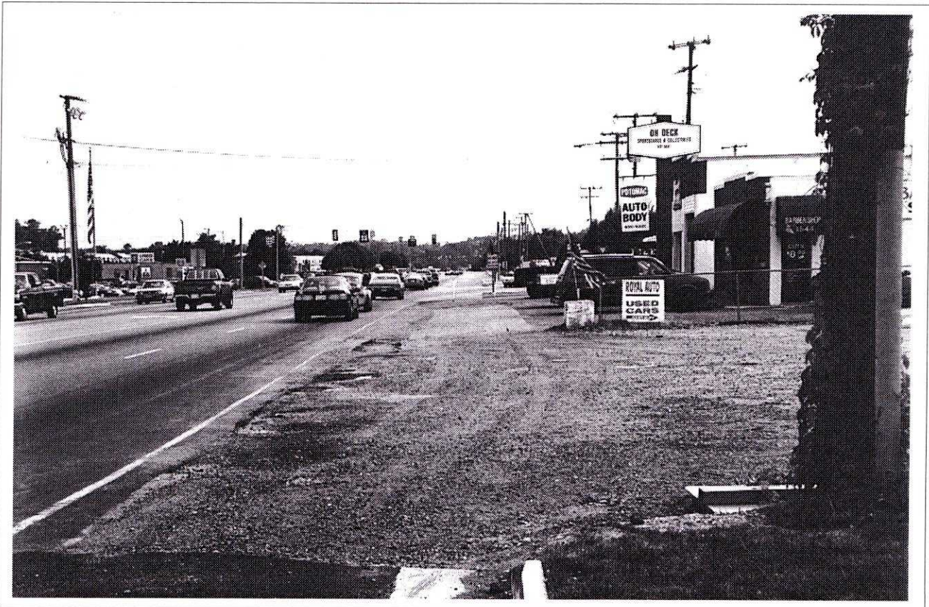
Lack of access control and lack of a consistent road edge treatment contribute to a negative image due to poor appearance and numerous traffic conflict points.
