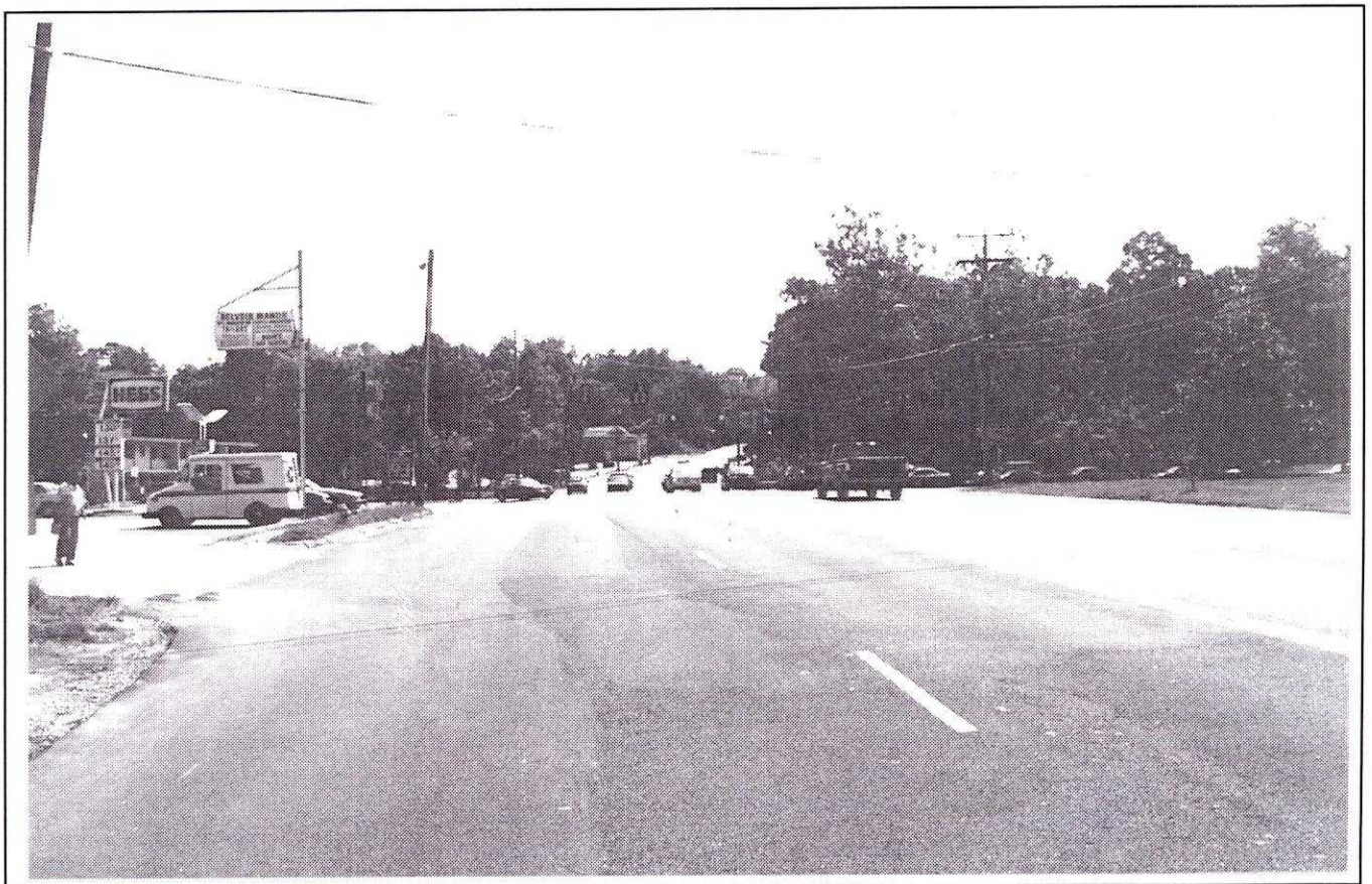
View looking north on Route 1 toward Backlick Road and Tulley Gate at Fort Belvoir
