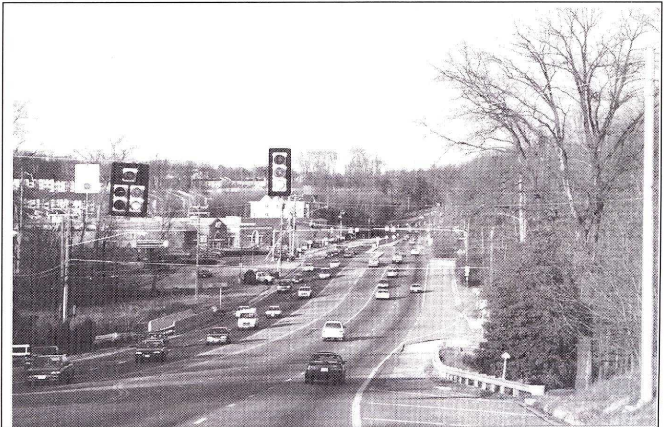
View looking north on Route 1 toward Armistead Road in Lorton
