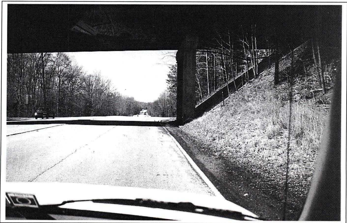
Fixed objects near the roadway, such as the bridge pier shown here, present potential safety hazards.
