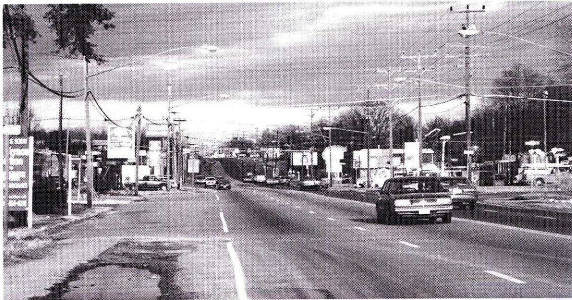
Most of Route 1 has received only spot intersection and frontage improvements over the last 30 to 40 years.
