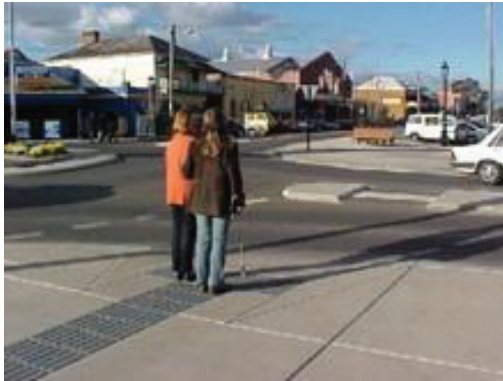
Figure 31: Good elements for pedestrians: reduced crossing distance, cut in median, tactile warning strip in curb cut
