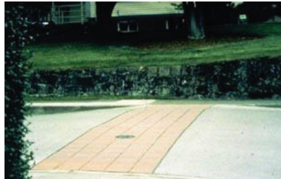
Figure 37: Raised crosswalk with distinctive surface provides visibility and slows vehicles
